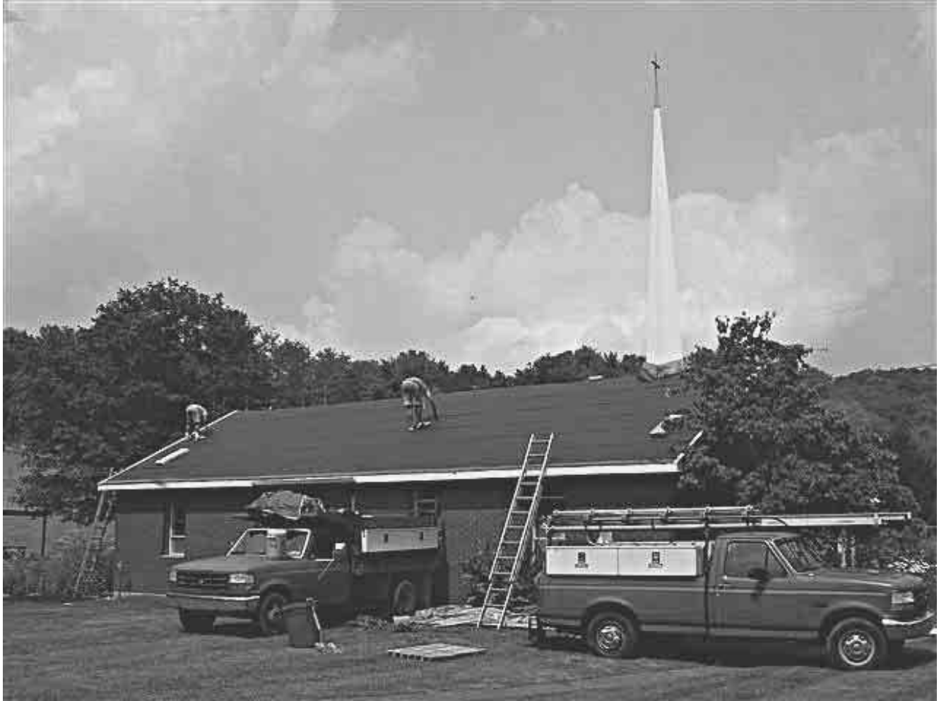
Our NEW ROOF being installed
